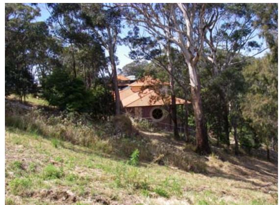
New dwelling under construction east of the site (Source: RDM)
